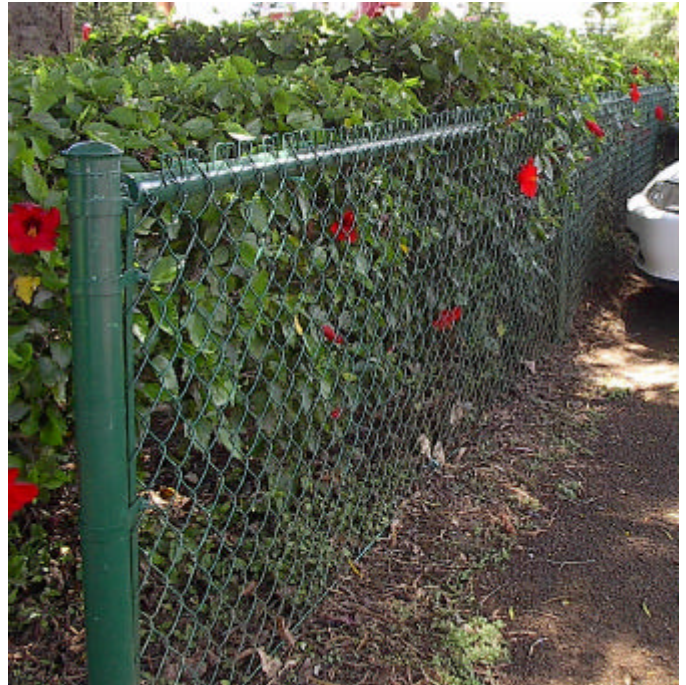
View (2) - Prince Albert Park new chain link fence
